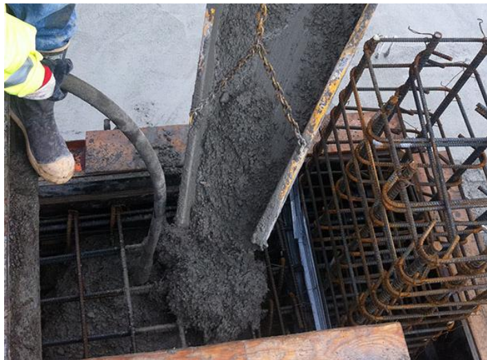
Figure 6: Casting of fiber reinforced concrete coupling beam in The Martin building
