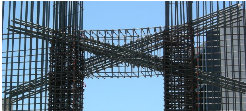
Figure 1: Diagonally reinforced earthquake-resistant coupling beam
