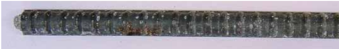
Figure 11 – Typical corrosion at initiation on conventional steel bar
